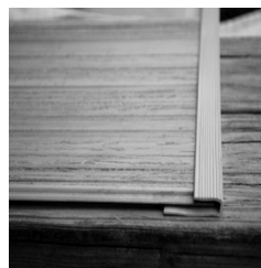
Side Edge Use the Multi-Trim Side Edge and remove the bottom part to obtain the Side Edge
